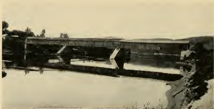
OLD WOODEN CHESHIRE BRIDGE BUILT ABOUT 1800
